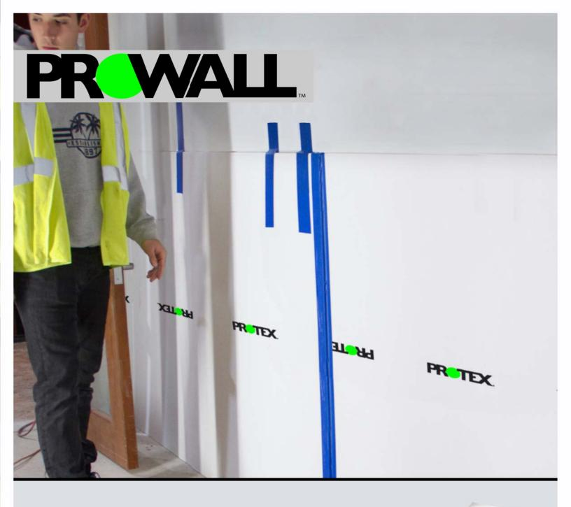
PROWALL - Heavy-duty temporary wall protection panels.
