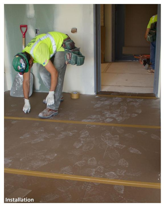
PROBoard™ 24's Tru-Lay Flat™ sheets made moving and installation much easier and faster. Using the GaffGun™ made installing the 26.2 miles of KTape™ seam tape extremely easy and fast.
