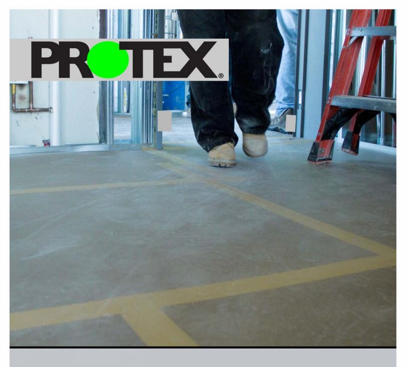
PROTEX - Standard-duty, Fire Rated, temporary job-site surface protection sheets.
