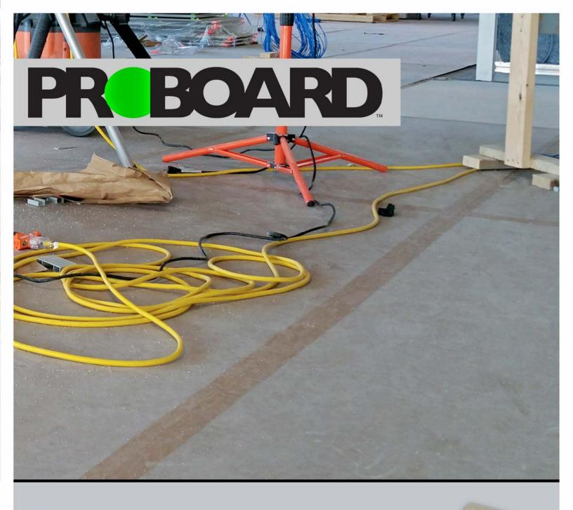
PROBoard - Heavy-duty, Fire Rated, temporary job-site surface protection sheets.
