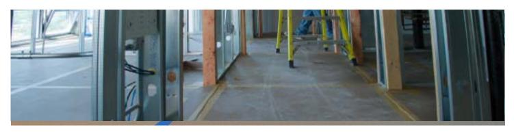
PROBoard™ - Heavy-duty temporary surface job-site layout board protection sheets that provide superior spill, impact and puncture resistance for more demanding projects.
